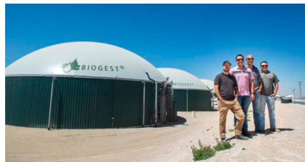
Picture: BIOGEST® PowerDigest biomethane plant, 184,000 MMBTU/year (585 Nm 3 /h), Oak Valley, South Dakota, US
